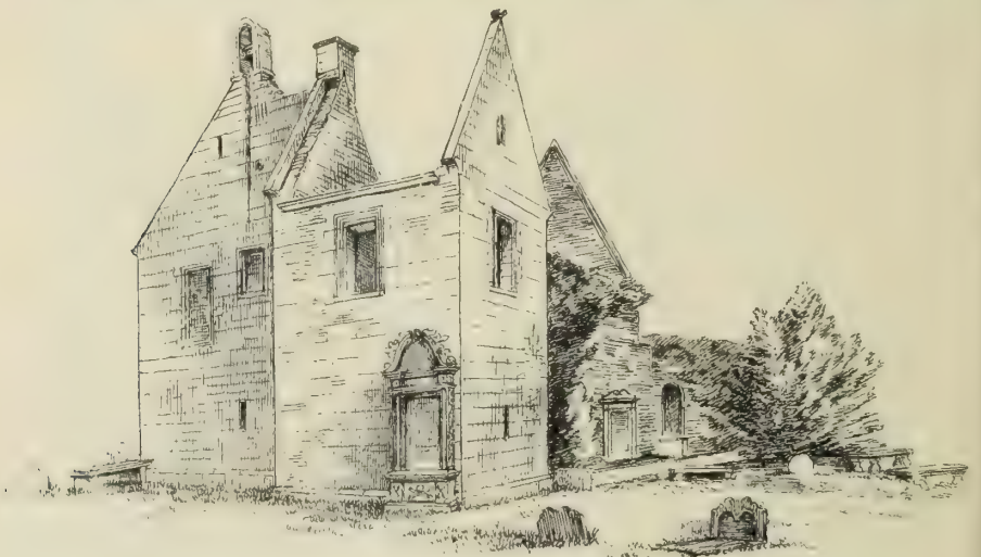
FIG. 1521.—St. Bridget's Church, Dalgety. View from South-West.
